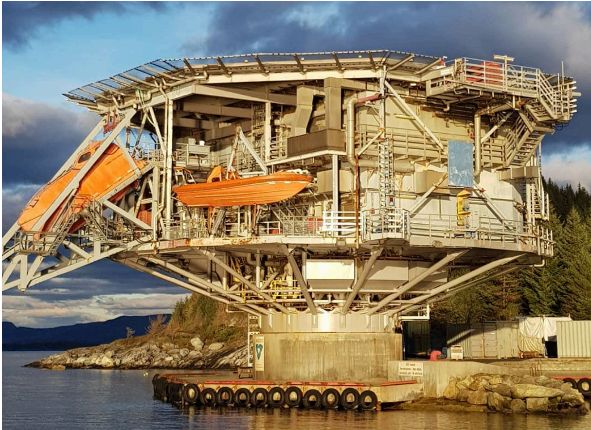
Figure 2 The Offshore Structure at Tau Autonomy Center.
